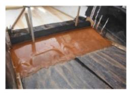
Siltworm's unique composition of a rolled fabric netting filled with a proprietary blend of 100% recycled, kiln-dried wood fiber allows water to flow through as sediment remains behind the effective barrier at the end of the water flow, as pictured.
